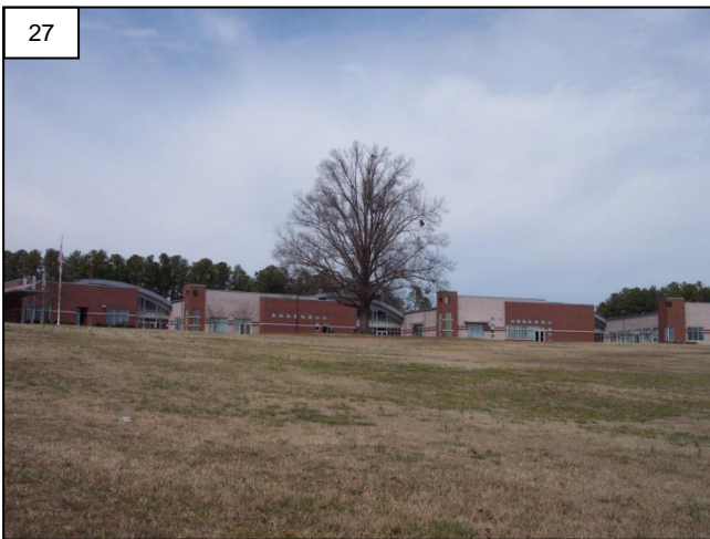
Butner-Stem Middle School on the north side of D Street west of 24 th Street.
