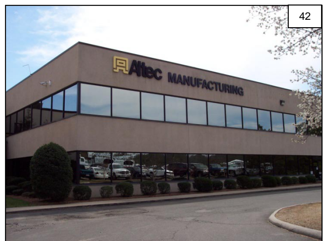
Altec Manufacturing facility on Falling Brook Drive west of NC 56.
