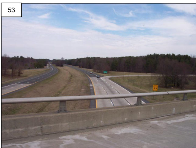
Looking north along I-85 towards Butner from the US 15 overpass.
