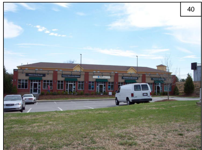
Commercial development on the east side of NC 56 along Capitol Drive.
